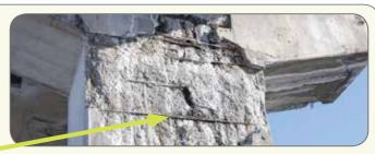
Swelling of steel reinforcement due to rust buildup has broken away the concrete cover, exposing the steel and making it even more vulnerable to corrosion, threatening the integrity of the entire structure.
