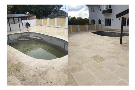
The travertine pavers around the pool required sealing with DRY-TREAT 40SK™. This is because the porous, softer stone is more susceptible to efflorescence and salt spalling. These problems are not only unsightly, but can damage the stone.
